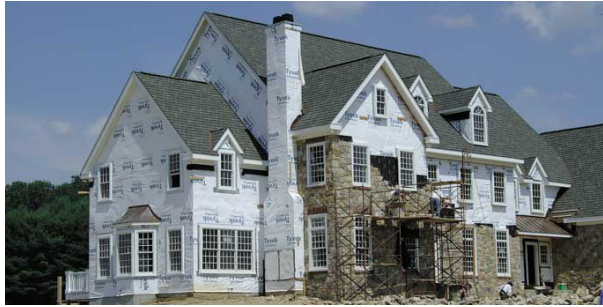
Tyvek in white and brick cladding in brown
